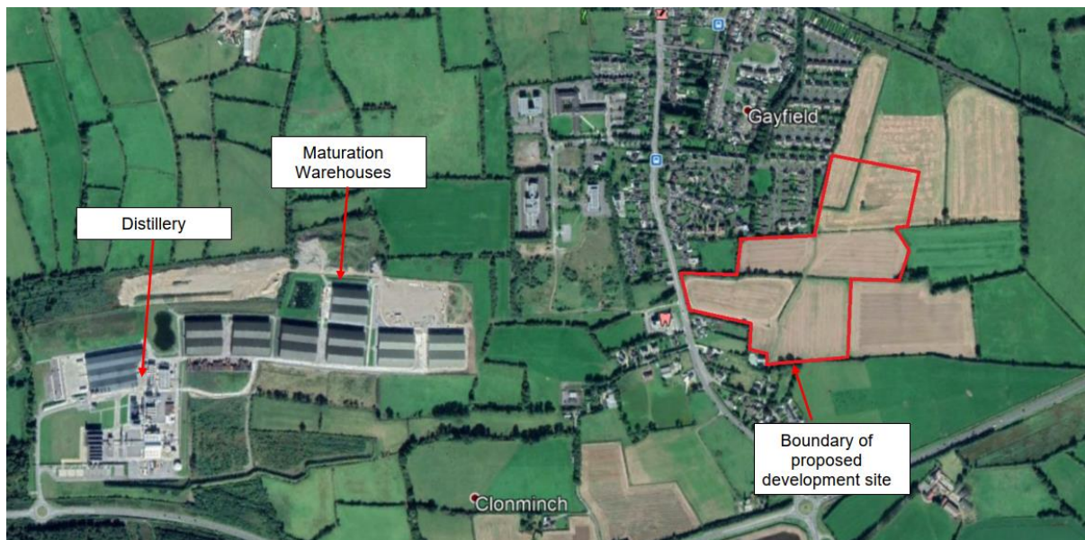
Figure -4.10 – Approximate application site boundary in relation to William Grant & Sons Distillery
